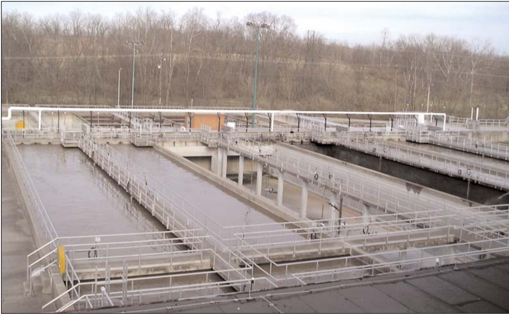
The West Hickman Creek WWTP fermentation zone created by conversion of primary settling tanks has a BPR volume of 1.448 million gallons. Hydraulic retention time (HRT) at 40% RAS rate is 44 minutes.
